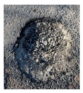
Step 2, use a gas or electric blower to blow out all the lose material from inside the hole
