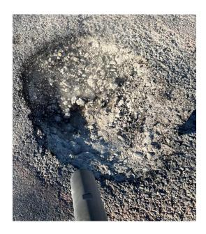
Step 3, Open a bucket of Asphalt Bonding Agent called "Tack" (HomeDepot.com Asphalt Bonding Agent SS-1H Tack Coat (\$50.92 each) and using an old stiff bristle broom, dip that broom into the "tack" and thoroughly "paint" the inside of the hole. Make sure that you cover the upper sides of the hole and even over the top of the pothole.
