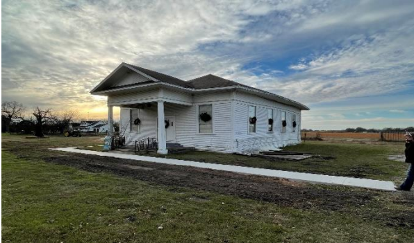
Special thanks to HR Dirt Works for installing the new sidewalks at the Camp Ground Church seen here.
